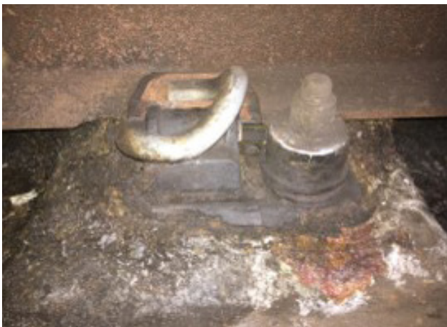
Corrosion to rails
